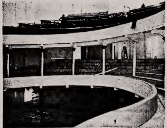
Work has been going on for six years. Interior construction began two years ago. This is a view of the orchestra floor, the dress circle (center) and the family circle (top).
